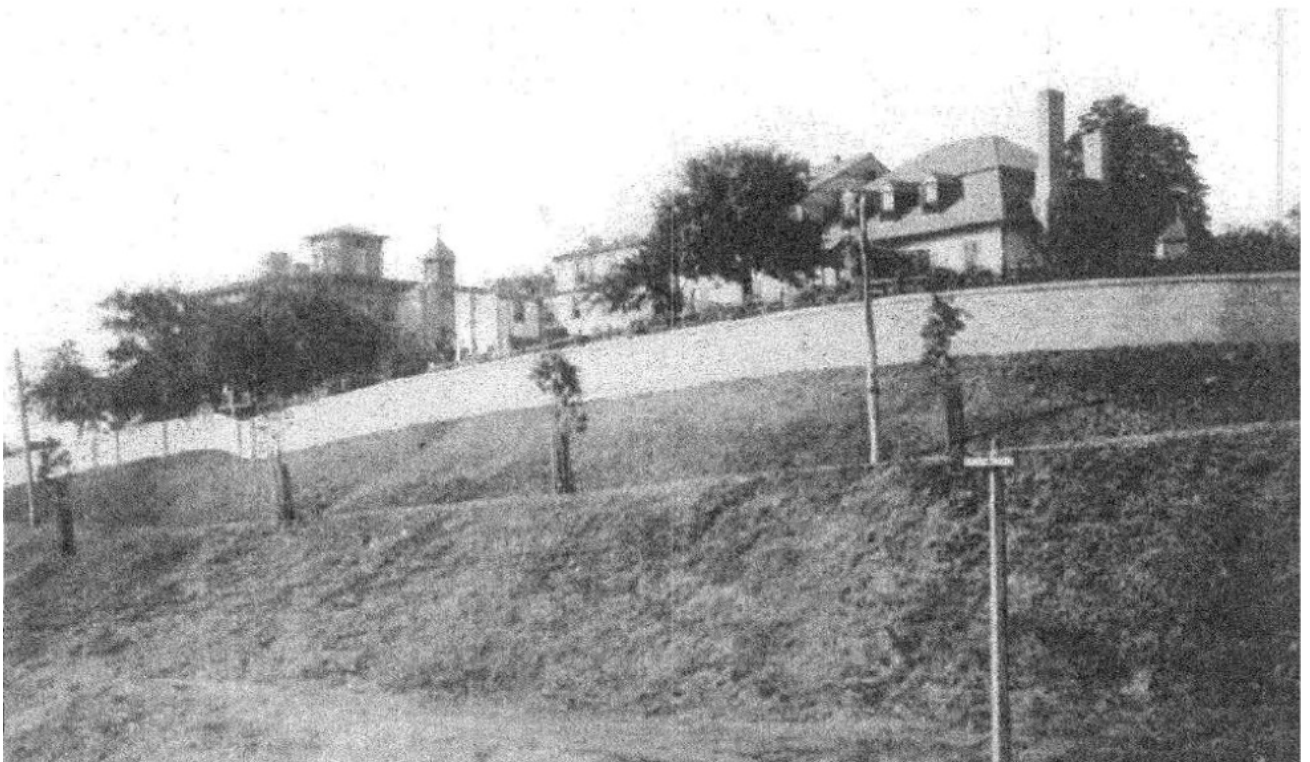
(The brick wall constructed around 1909 – photo taken from southeast)
